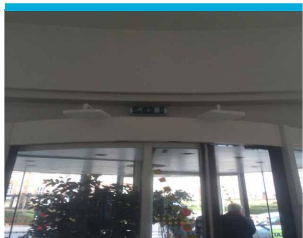
Figure 4: RFID readers installed at doors in the hospital.
